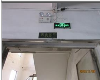
External photo(s) of the production unit(s) NO-19 Exit sign and emergency light.JPG
